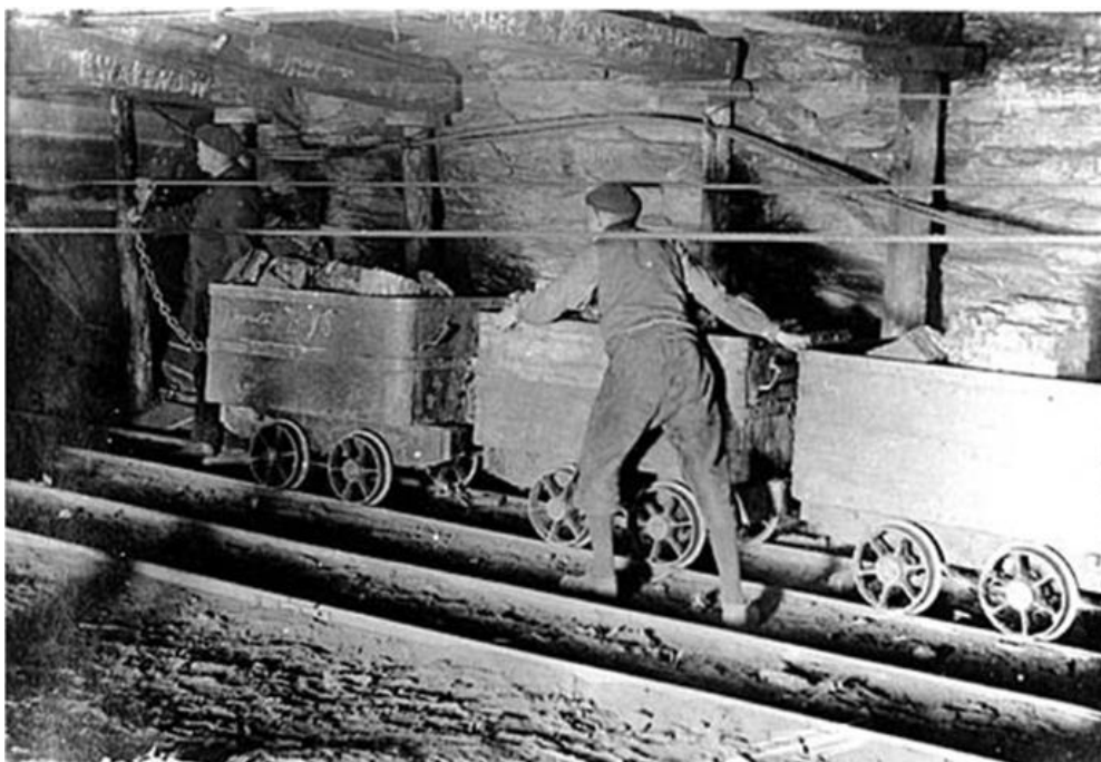
These two old photographs dated around 1900 show two haulage systems that were still in use at Kemball T.C. in 1957. Above this man is coupling a wagon to the haulage rope by way of a "Clip" below these men are using a lashing chain to attach the wagons to the rope.
