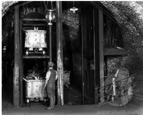
Top: men in one of the decks of a cage, Btm: coal going up the pit in a two decked caged
