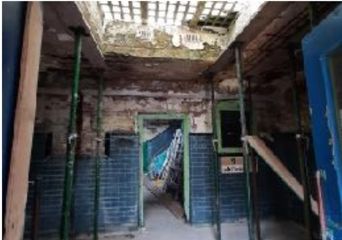
We have managed to secure a grant to stabilise the entrance to the Pit Head Baths and work has started. They have removed all the old wooden boarding which was 'holding' the roof up, which was suffering from the metal tie bars corroding and bring down the concrete. It has already transformed the place and exposed a skylight. The steels are NOW in and the next phase will be the roof and then a wait for the place to dry out....
